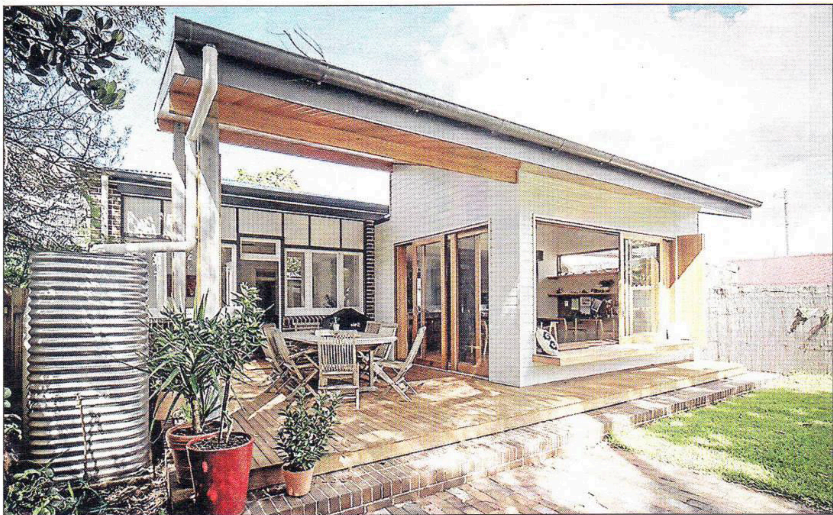
Mackenzie Pronk Architects' reinvention of the old double-fronted house straddles both inside and out, with an oversized retractable window system connecting the dining-kitchen area with the garden.
