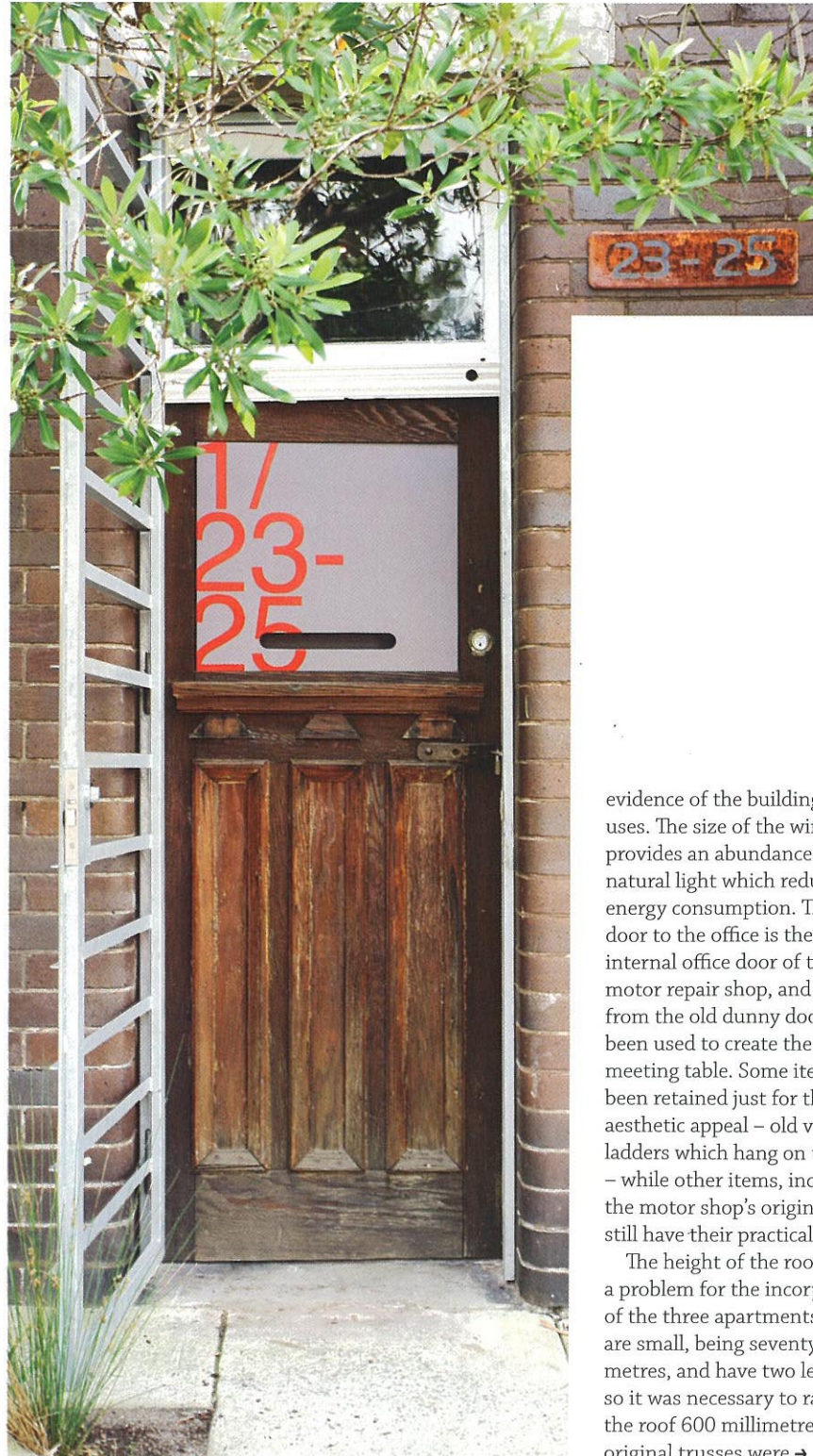
The office door of the old motorshop has been repositioned as the front door of the office.
